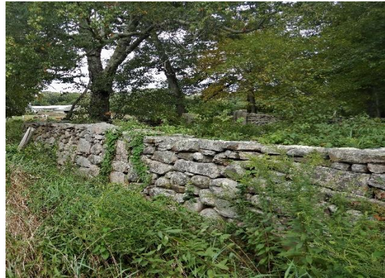
Roadside West Wall
